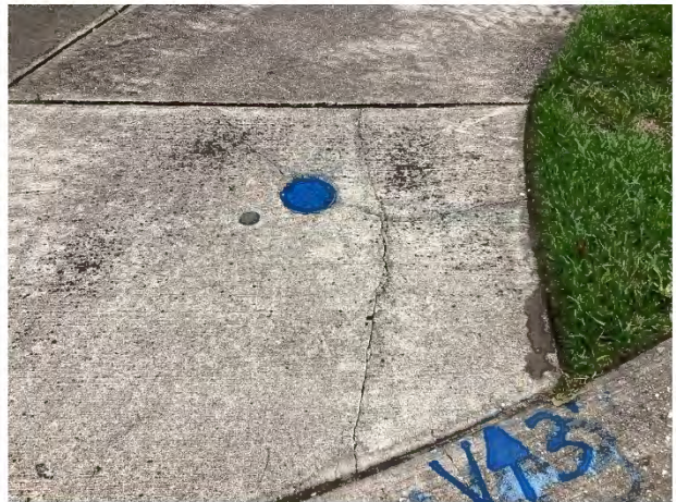
Sidewalk cracks
