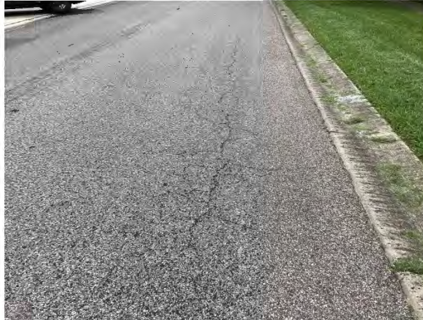
Pavement cracks
