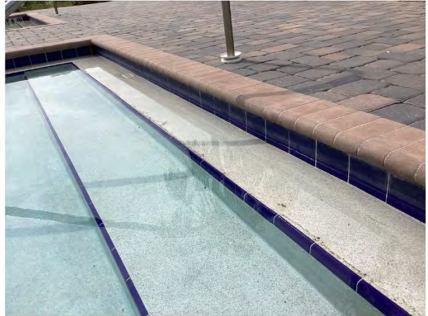
Pool plaster finish with tile perimeter
