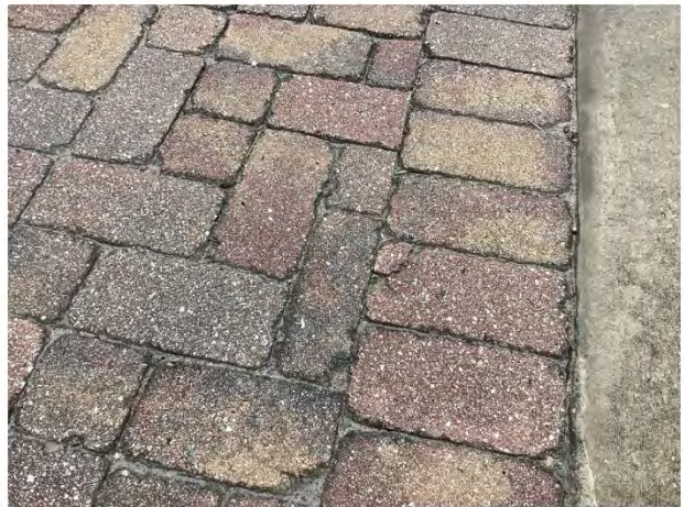
Paver cracks
