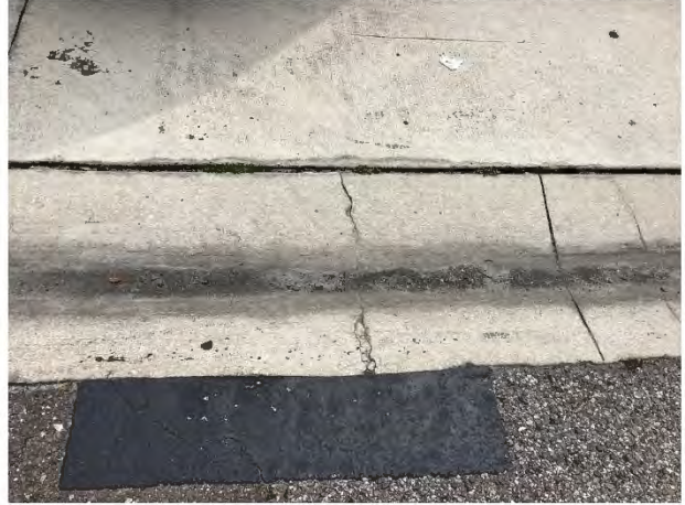
Concrete cracks
