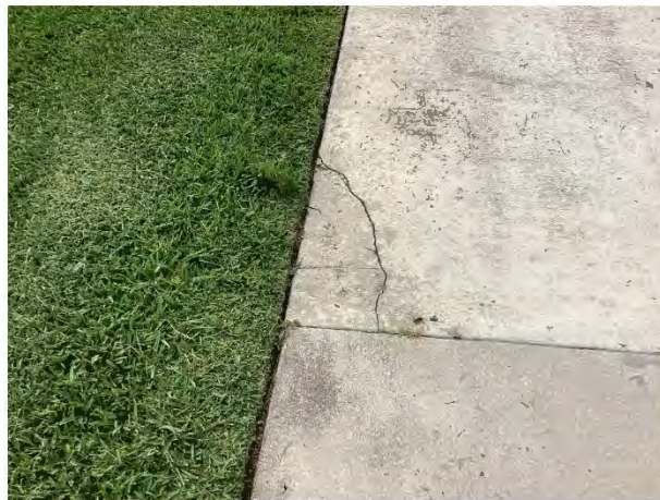
Sidewalk cracks
