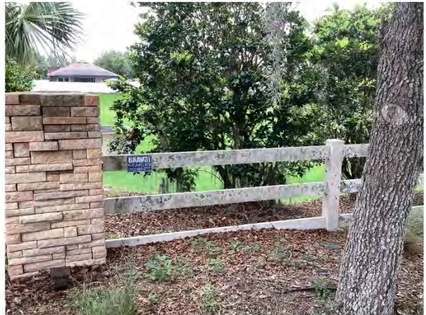
Fence finish deterioration
