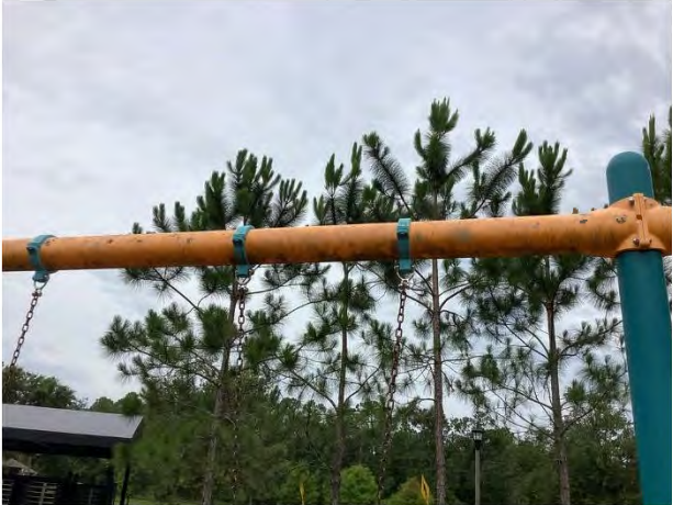
Equipment finish deterioration
