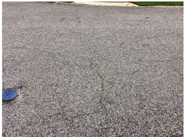
Pavement cracks
