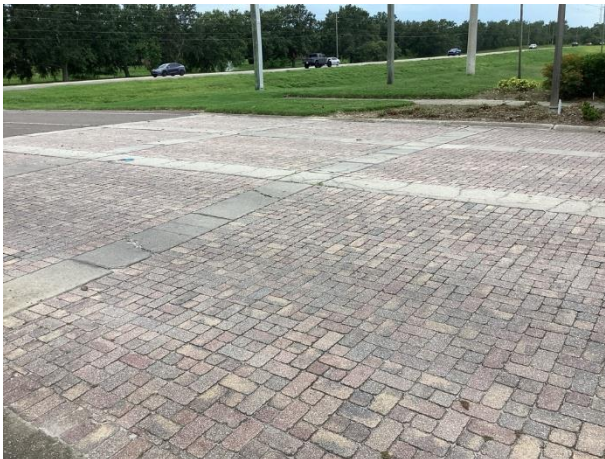
Masonry pavers overview
