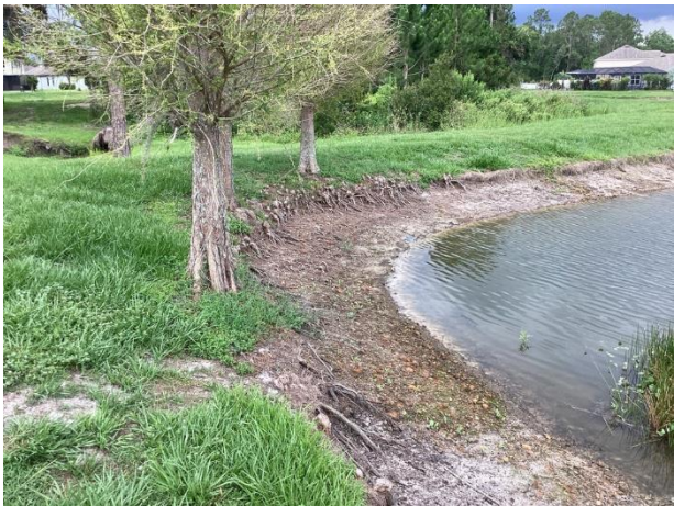
Minor shoreline erosion
