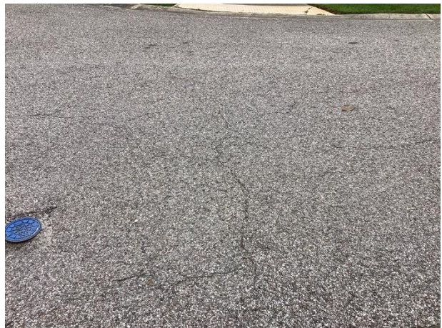
Pavement cracks
