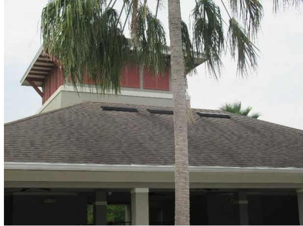
Clubhouse asphalt shingle roof
