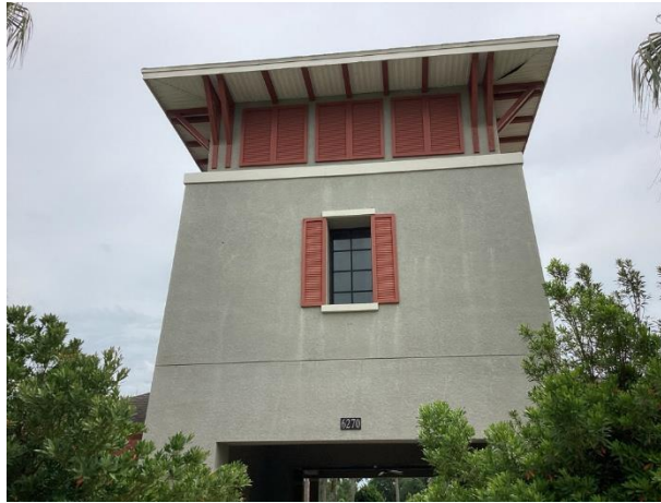
Stucco wall finishes
