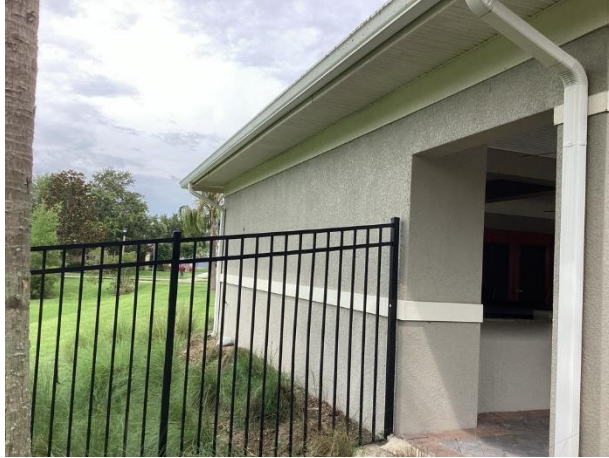
Stucco wall finishes
