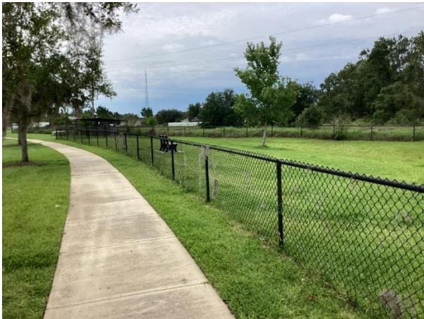
Chain link fence
