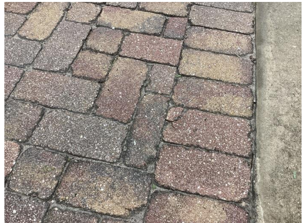
Paver cracks
