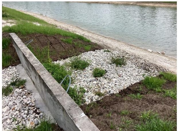
Shoreline remediation at pond control structure
