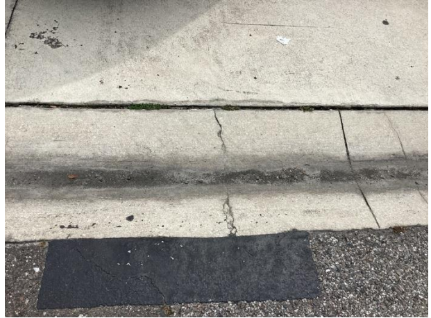
Concrete cracks
