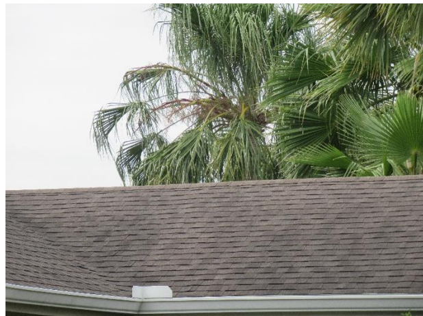
Clubhouse asphalt shingle roof
