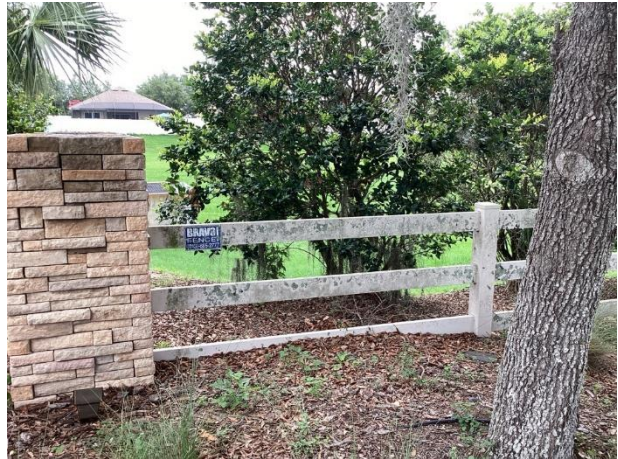
Fence finish deterioration
