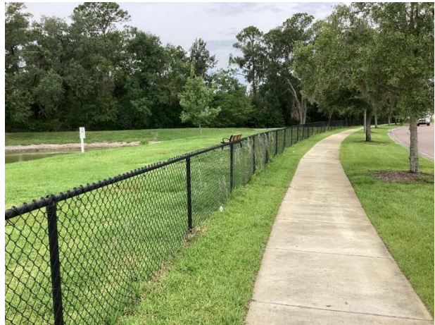
Chain link fence
