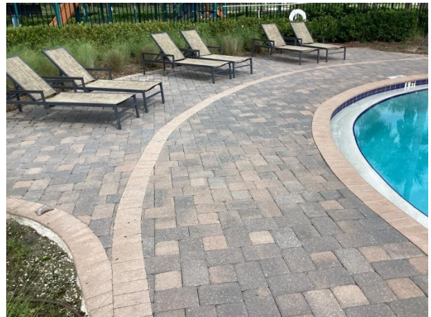
Paver pool deck overview
