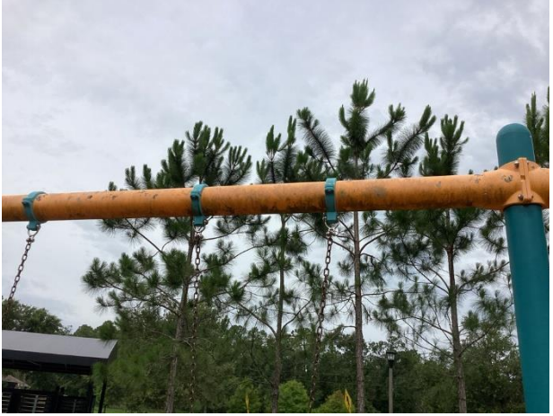
Equipment finish deterioration
