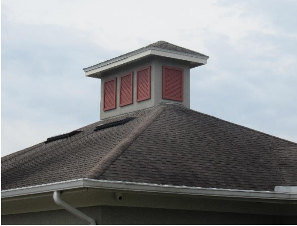
Clubhouse asphalt shingle roof
