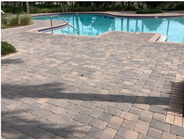
Paver pool deck overview
