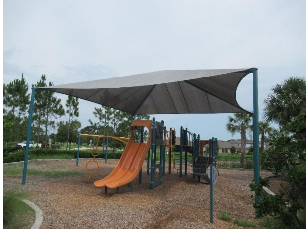
Shade structure overview
