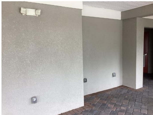
Stucco wall finishes
