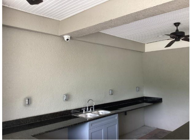
Stucco wall finishes
