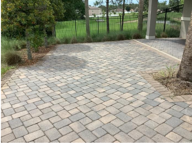
Paver pool deck overview
