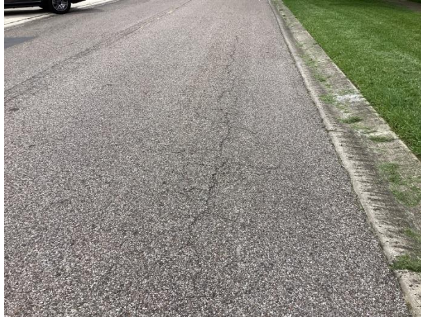
Pavement cracks
