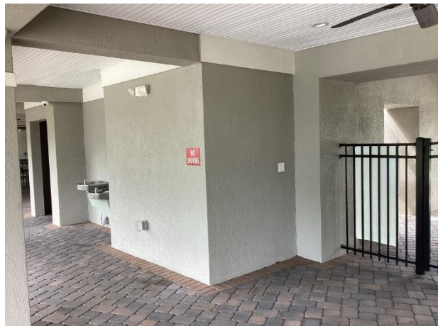
Stucco wall finishes
